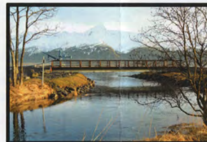
H. Scheffler Creek Bridge
