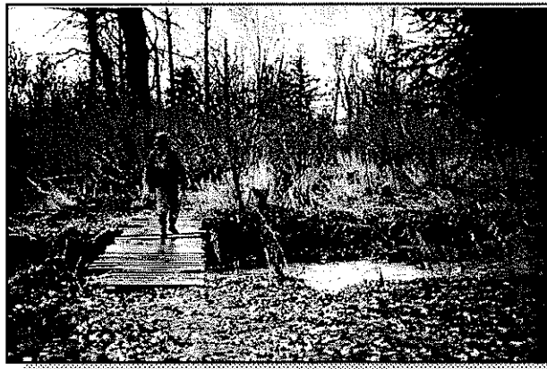
Bridge across California Creek.
