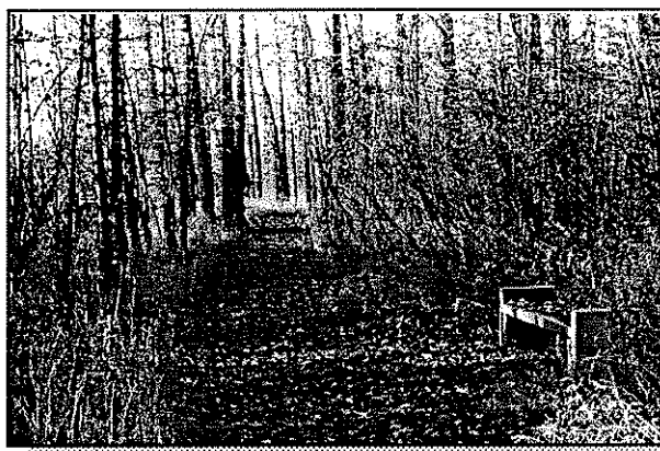
Packed granular stone trail developed by the USDA Forest Service and Ducks Unlimited at Moose Flats in the Portage Valley.
