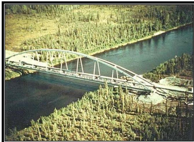
**Kuparuk River Bridge** Oil field traffic involving movement of large prefabricated building modules and drill rigs required bridges with live load capacities not previously envisioned. The Kuparuk River Bridge on the North Slope of Alaska was designed for a 2,300-ton live load. The solution used four steel box girders with a segmental concrete deck. Eleven general versions of this bridge type have been produced for mining and oil field projects.
