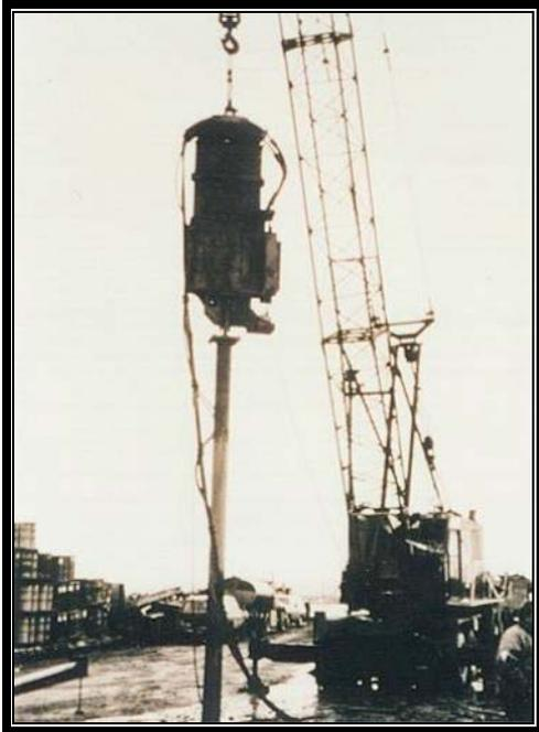
Research related to driven piles in permafrost and, following development, resulted in a patent and use of the thermally modified pilot hole technique for over 15,000 piles.
