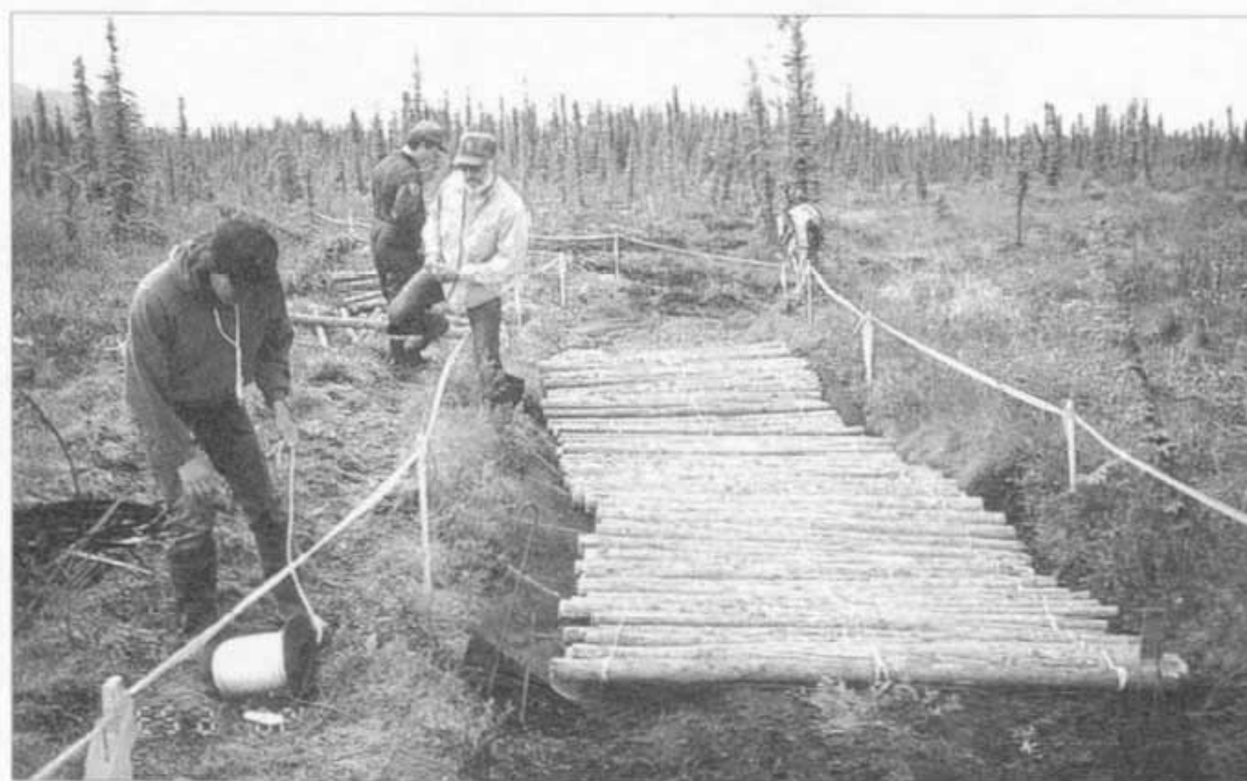
Crews applying corduroy to a heavily impacted trail section
