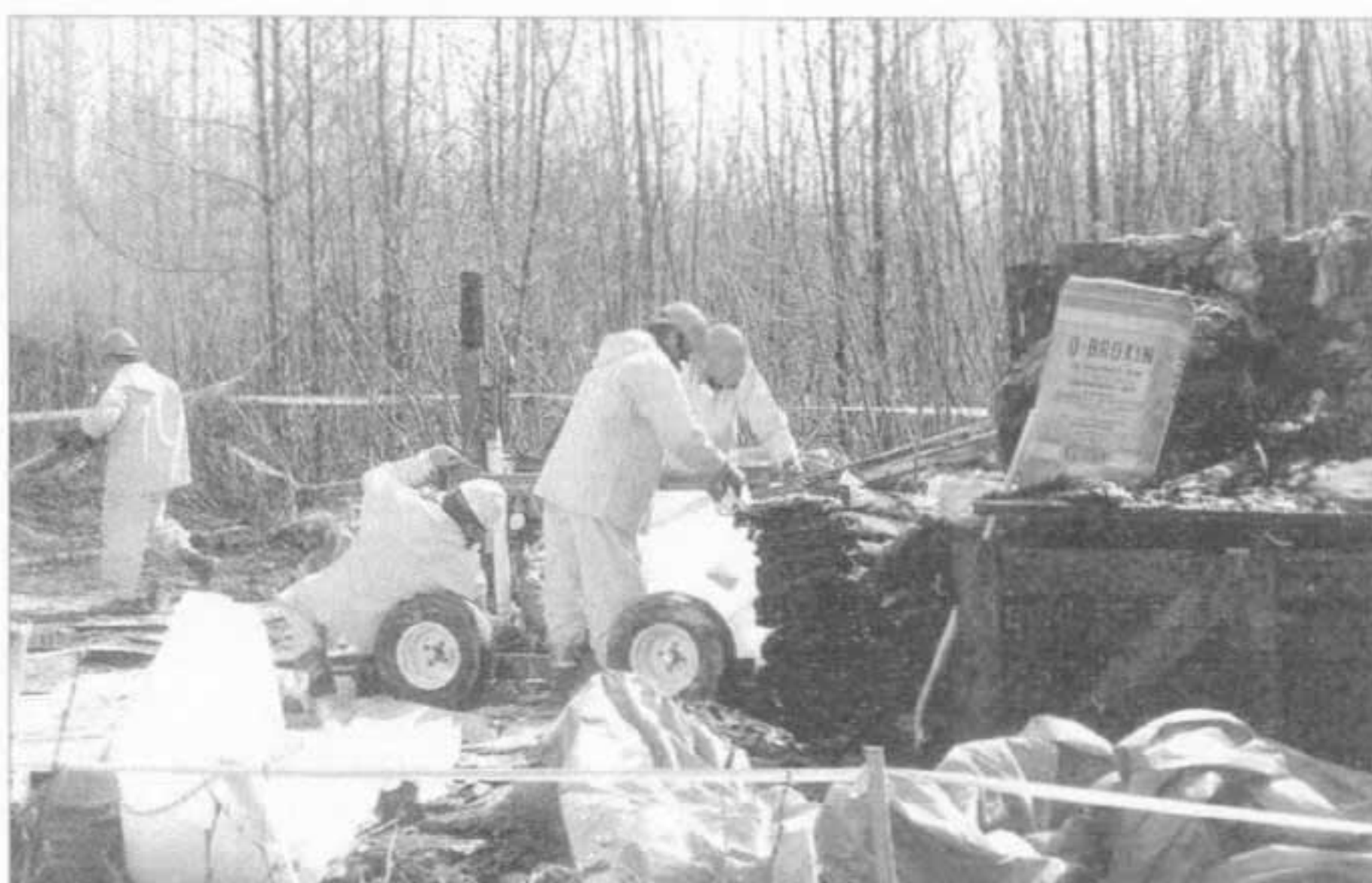
Crews removing hazardous materials at Sudden Stream
