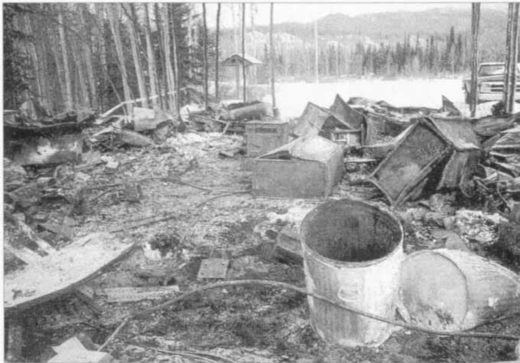
The Slana Ranger Station following the 1992 fire
