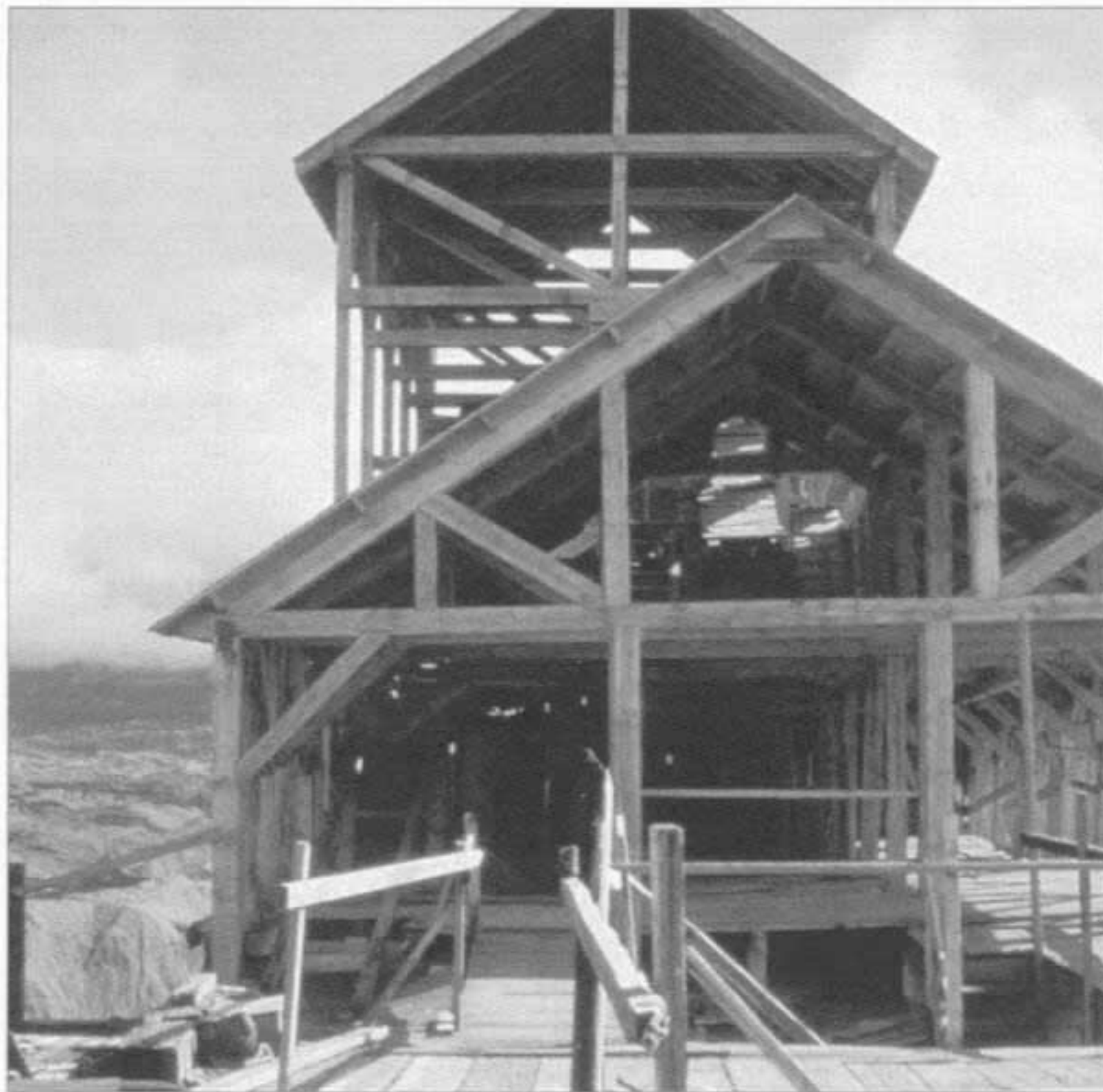
The mill's loading deck in 1993, following emergency stabilization by the Friends of Kennicott
