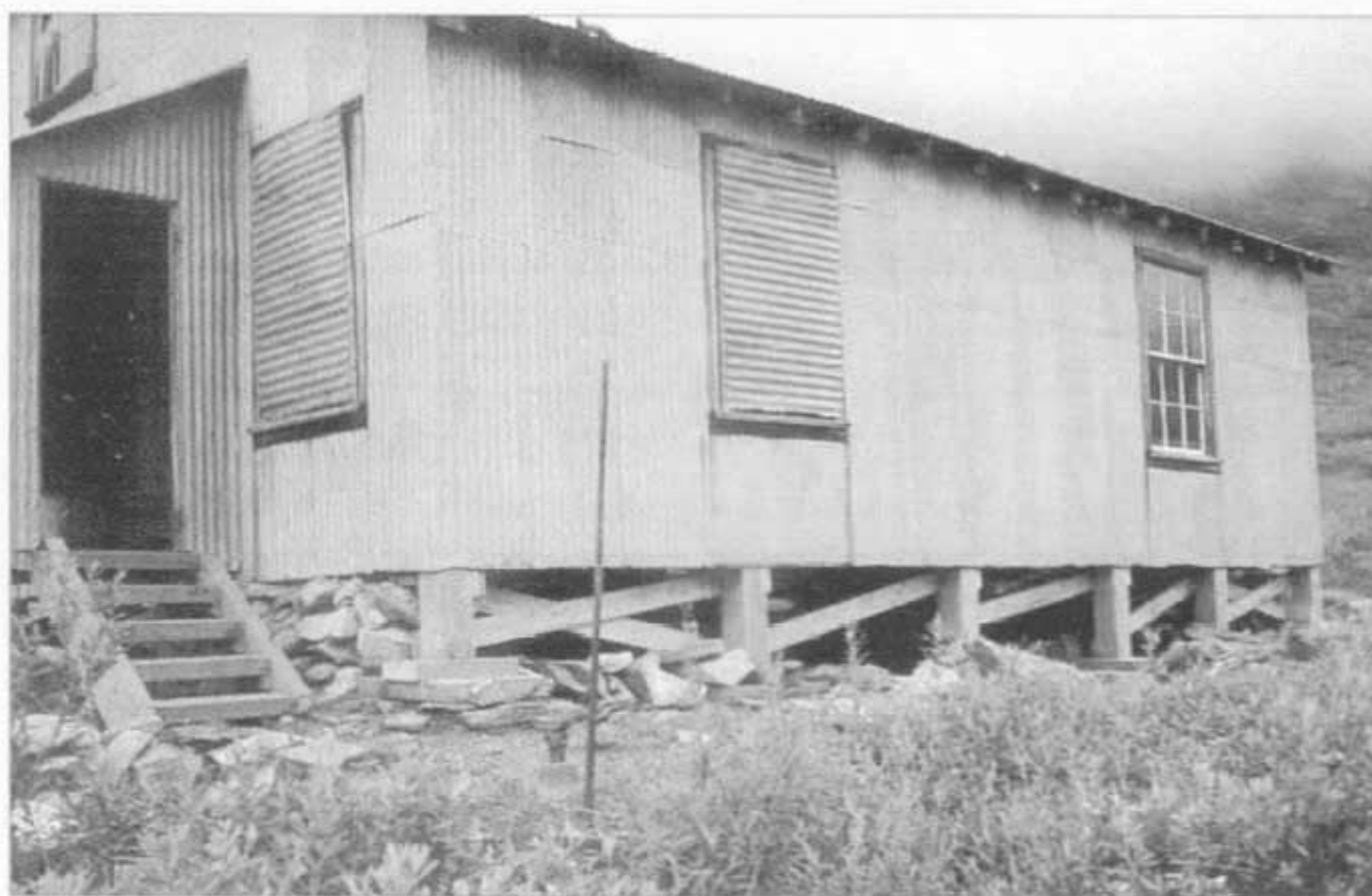
Park staff installed new cribbing under the Bremner bunkhouse
