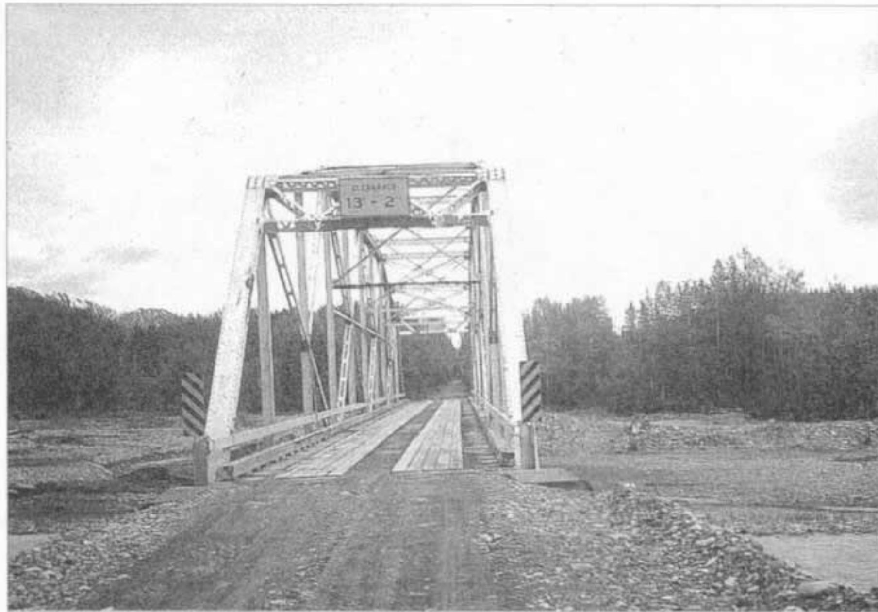
Recycled one-lane bridge over the Lakina River
