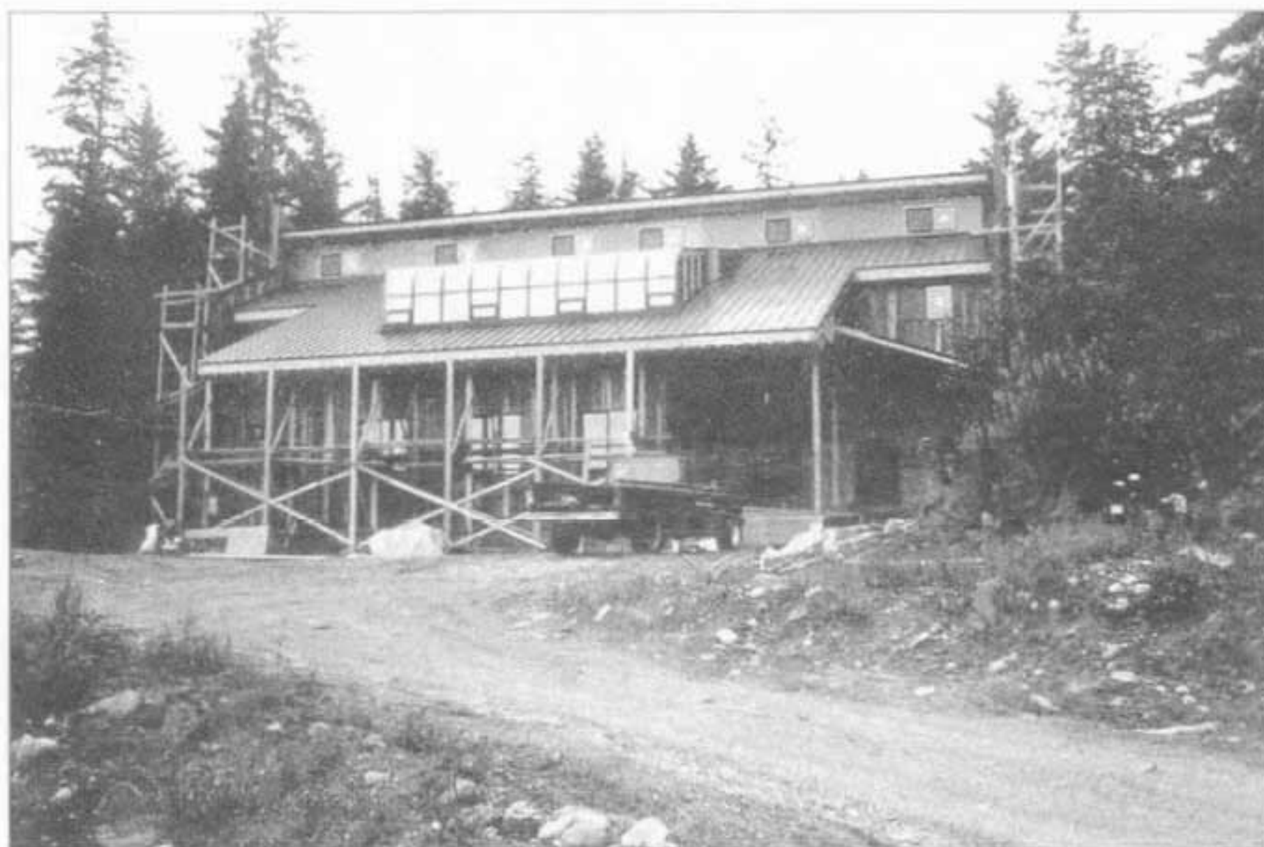
WRST's current Yakutat facility was constructed in 1993
