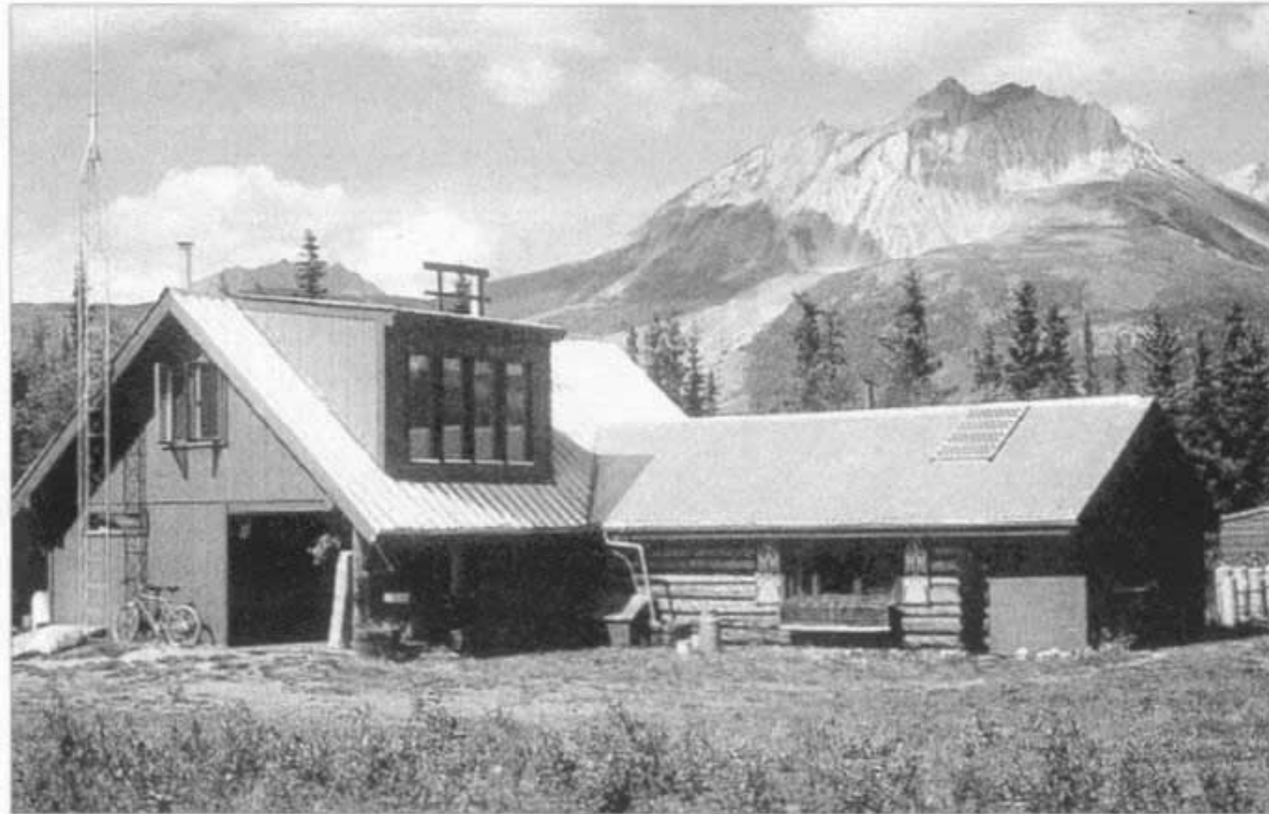
May Creek Operations Center
